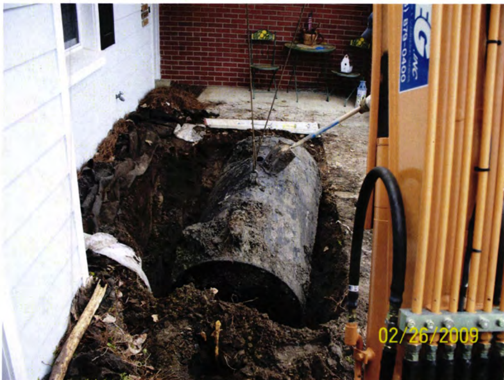
Picture 2: UST 116Banyan during removal.
